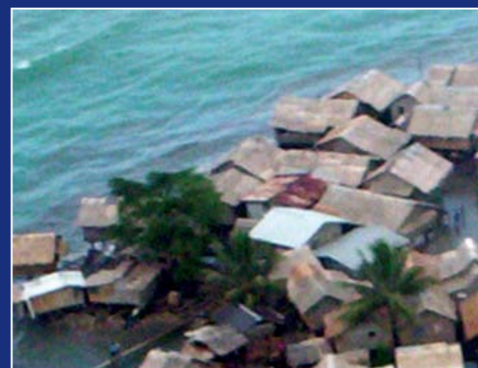
Figure 9. Flooding caused by a king tide on the artificial Island of Walande, Malaita Province.
